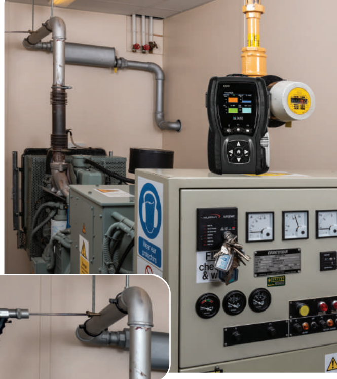
Gas Engine Testing with optional CHSP5 probe
